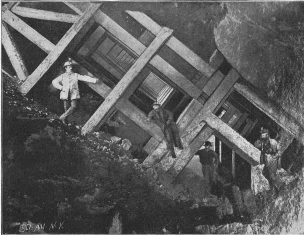
METHOD OF TIMBERING IN THE CALUMET AND HECLA COPPER MINE, 4,650 FEET BELOW GROUND.
