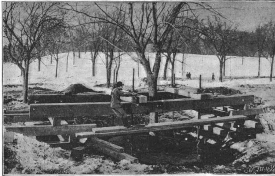
PREPARING TO RAISE A TREE.
