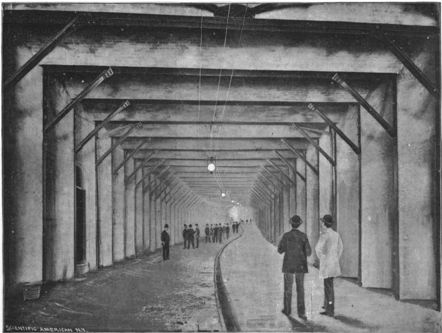
THE BOSTON SUBWAY—INTERIOR OF THE TWO-TRACK SUBWAY.
