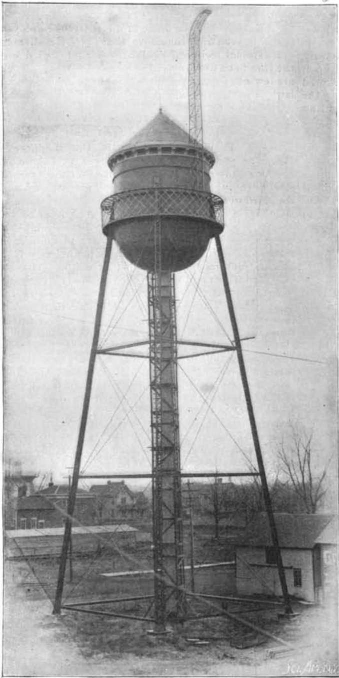
AN IRON WATER TOWER.
