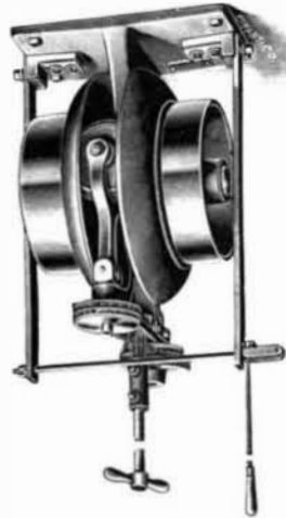
THE CUMMINGS' SPEED CONTROLLER.
