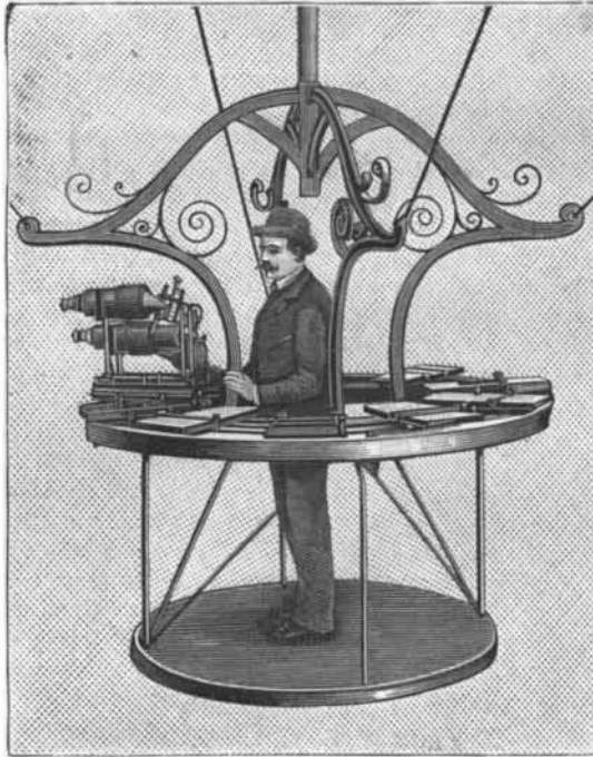
Fig. 3.—PLATFORM FOR THE OPERATOR AND PROJECTION APPARATUS SUSPENDED IN THE CENTER OF THE HALL.
