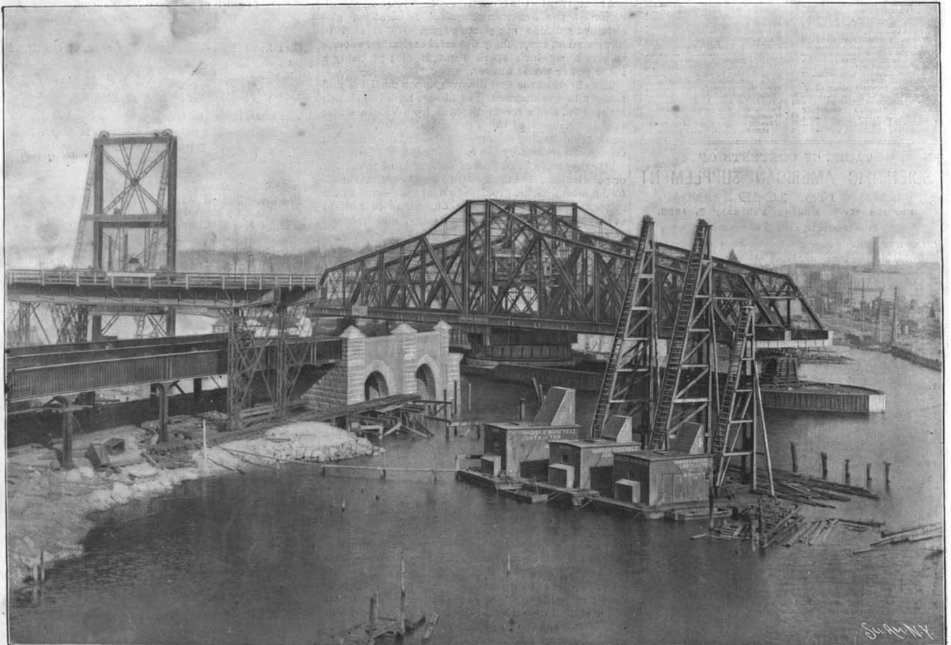
THE DRAW SPAN OF THE FOUR TRACK HARLEM RIVER BRIDGE, STONE ABUTMENT, AND ELEVATED ROADBED.
