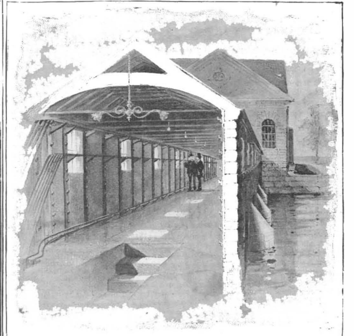
INTERIOR OF THE CABLE BRIDGE.
