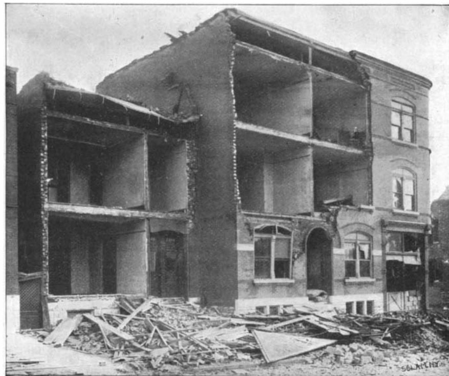
FRONT WALLS FORCED OUT BY VACUUM WITHOUT. LAMP LEFT STANDING ON TABLE ON SECOND FLOOR.
