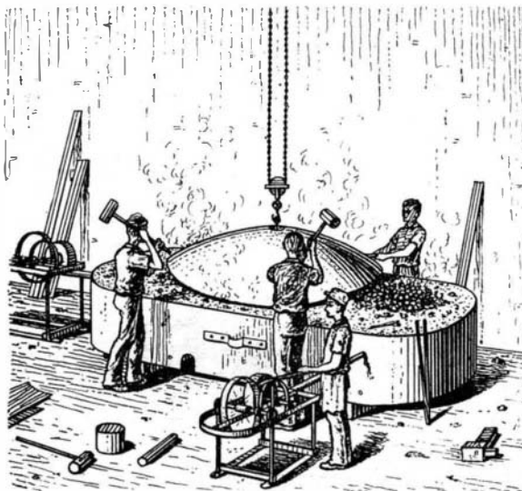
BEATING HEATED COPPER INTO SHAPE.
