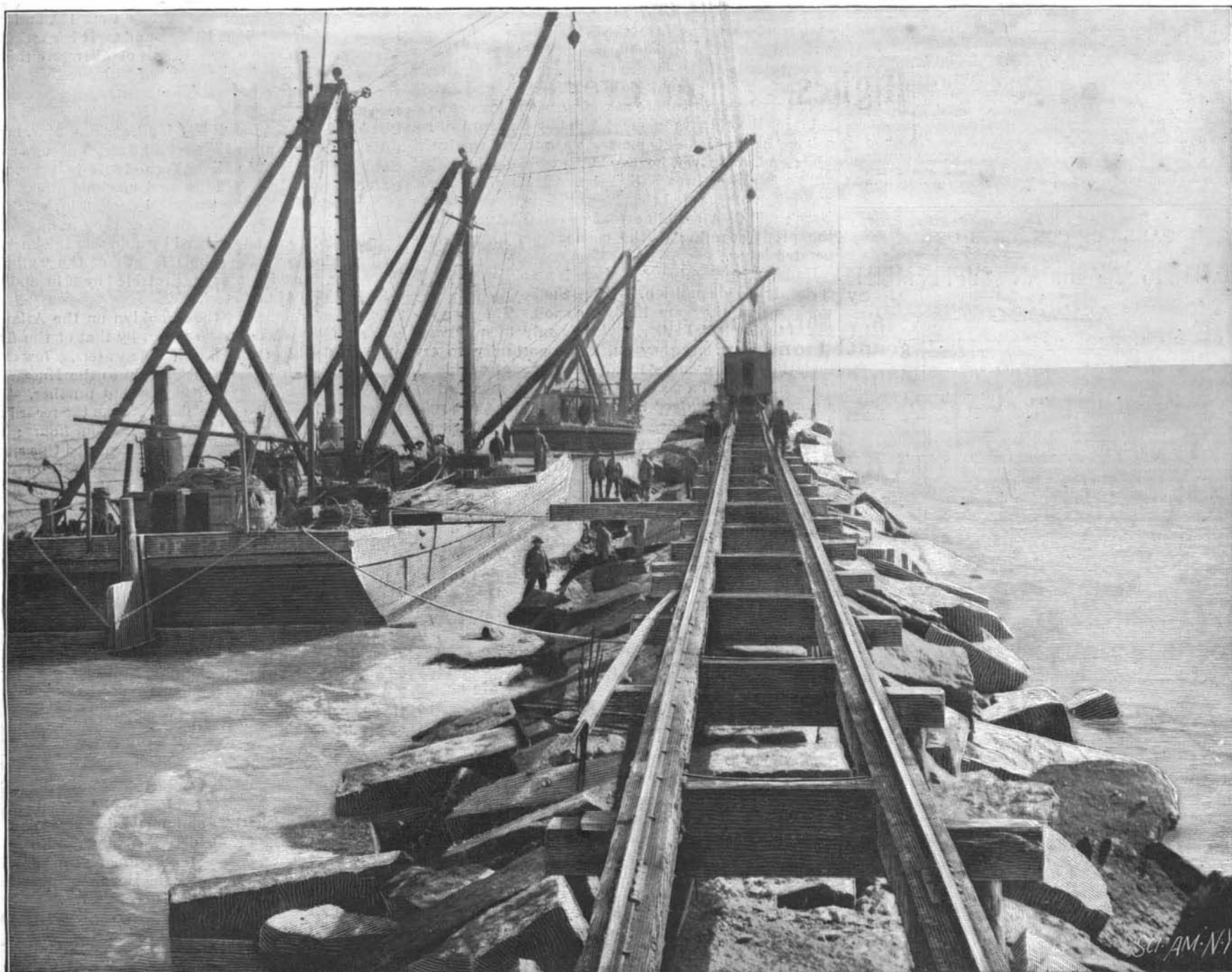
CONSTRUCTION OF JETTIES AT GALVESTON TEXAS.
