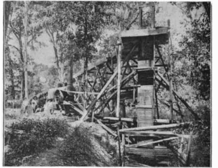
PUMPING ENGINE AND FLUME FOR A 1,000 ACRE RICE PLANTATION.
