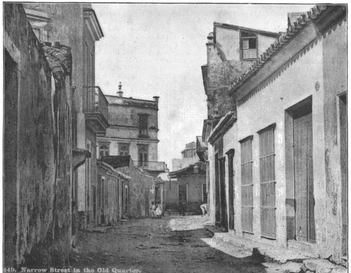
NARROW STREET IN THE OLD QUARTER, HAVANA.
