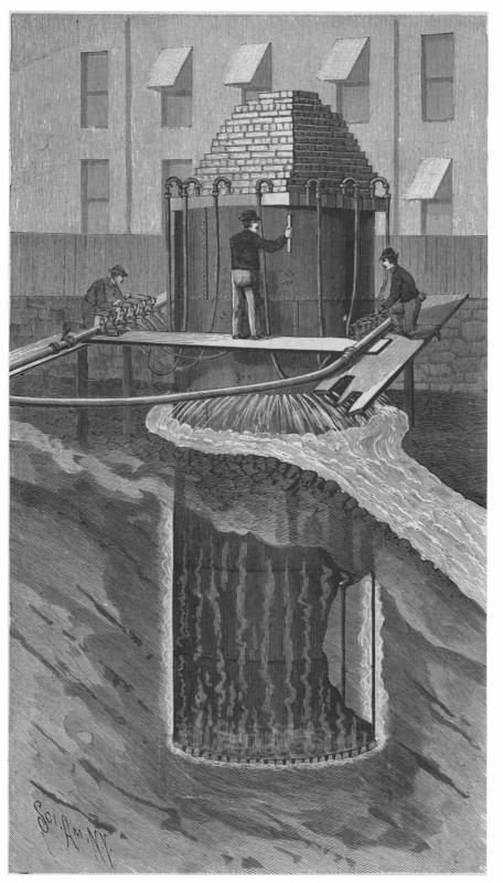
HYDRAULIC CAISSON SINKING FOR FOUNDATION PIERS.
