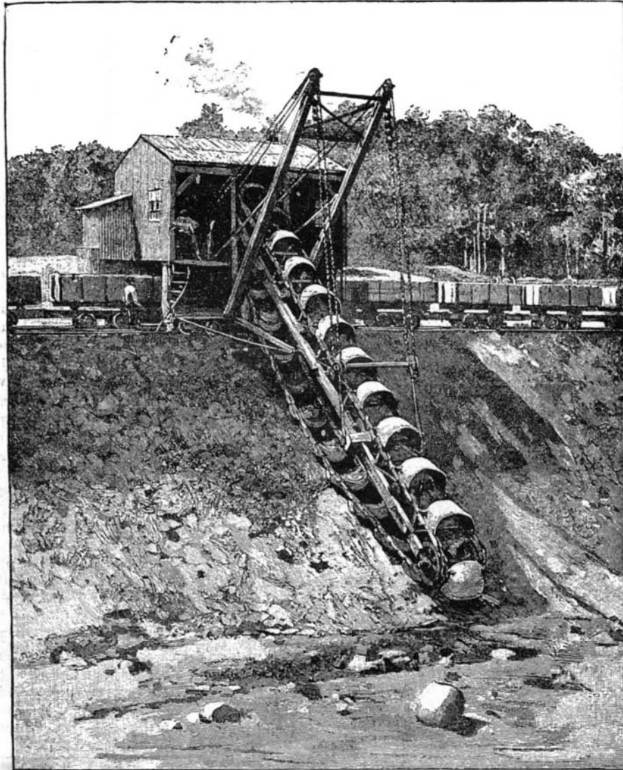
THE NORTH SEA CANAL—A STEAM SCRAPER AT WORK.
