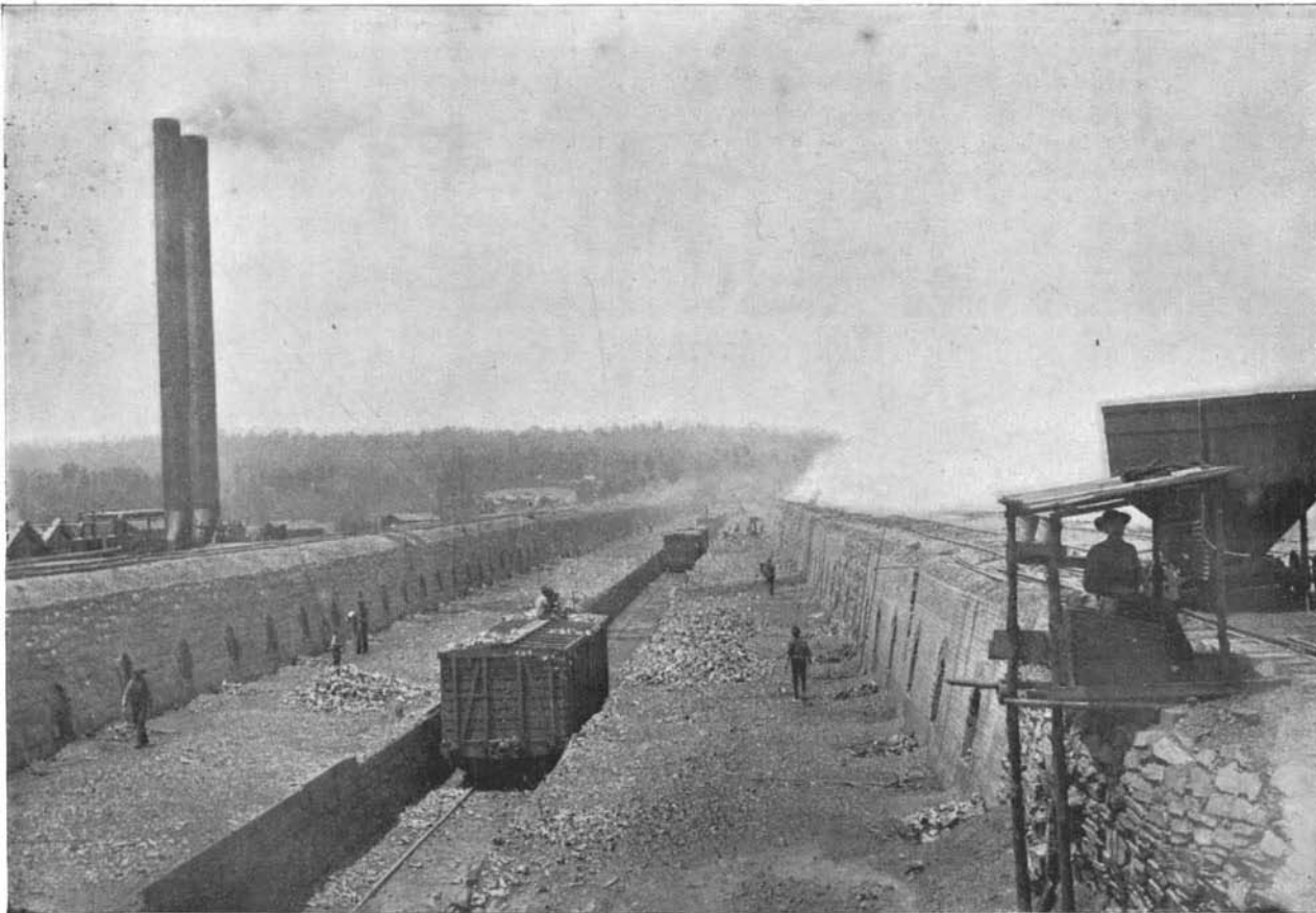
PLATT MINE COKE OVENS.
