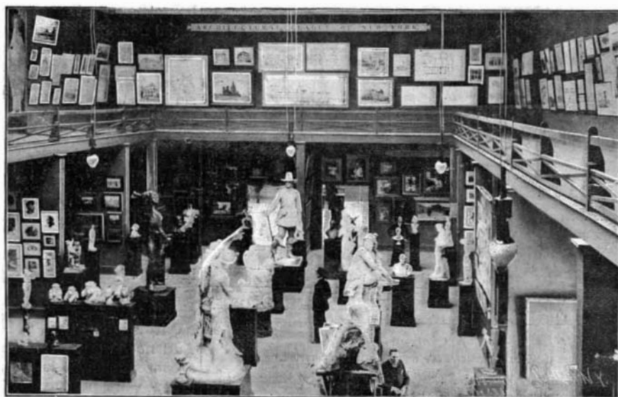
STATUARY HALL—FINE ARTS BUILDING.
