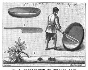
Fig. 5.—PREPARATION OF COLORED LACS. 1. Bowl. 2. Mixing tool. 3. Method of operating. 4. Branch of sumac, showing incisions.
