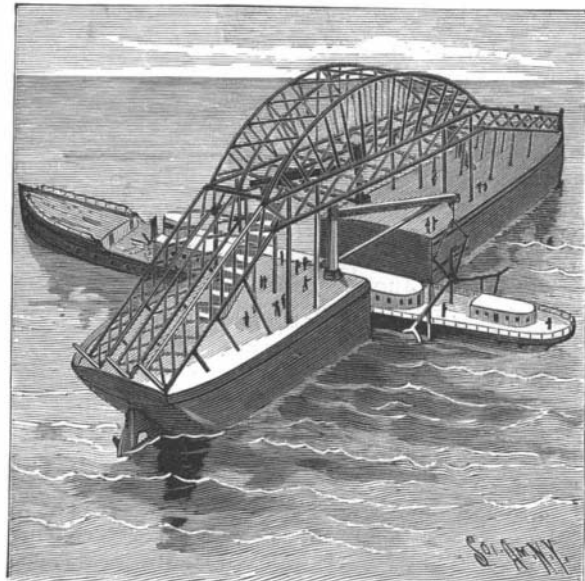
SCHON'S APPARATUS FOR RAISING SUNKEN VESSELS.
