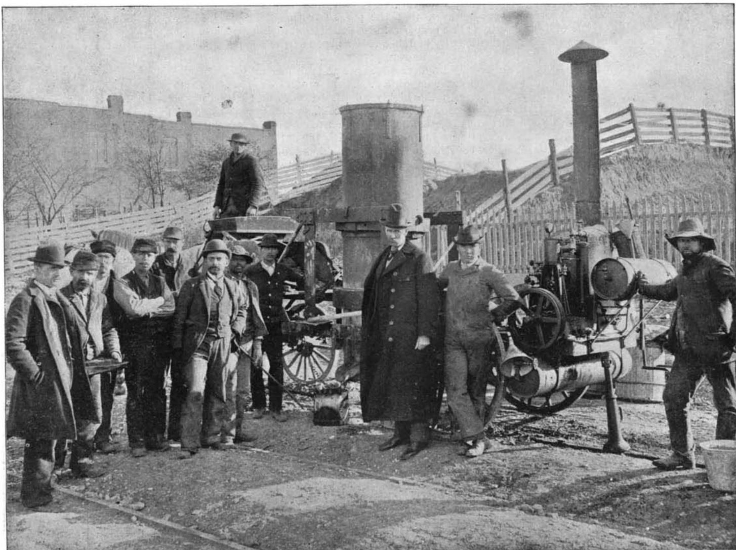
CASTING OUTFIT READY FOR WORK. CAST WELDING FOR RAILWAY RAIL JOINTS.
