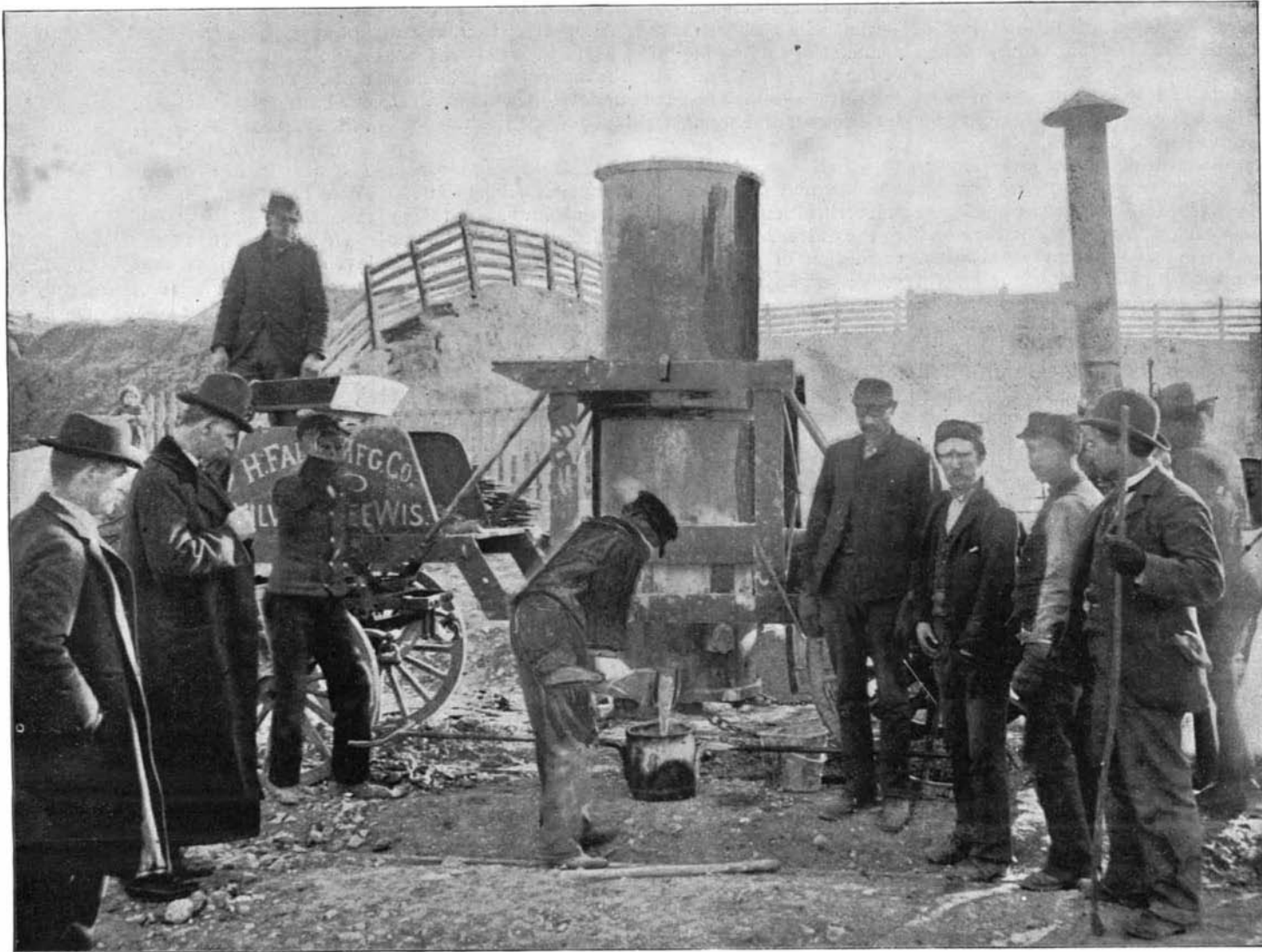
RUNNING THE METAL.
