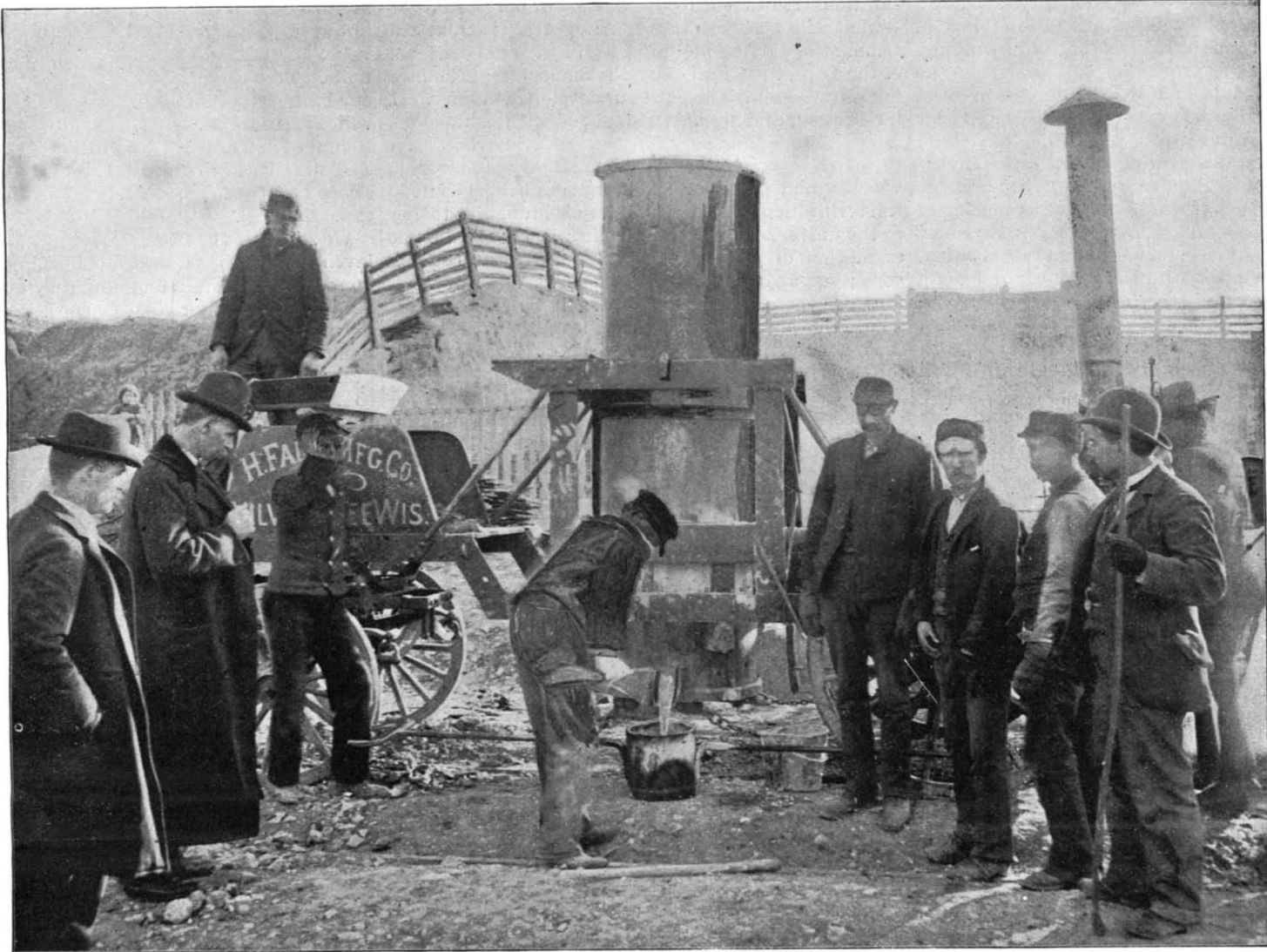
RUNNING THE METAL.
