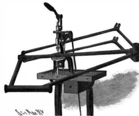
BICYCLE FRAME REPAIRING ON DRILL PRESS.
