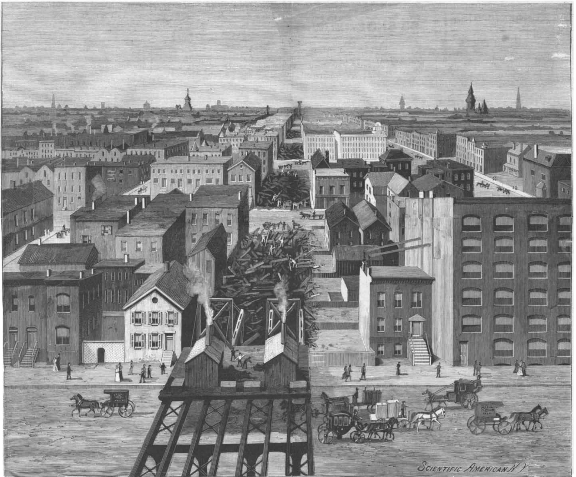
Moving the Normandie Flats.
