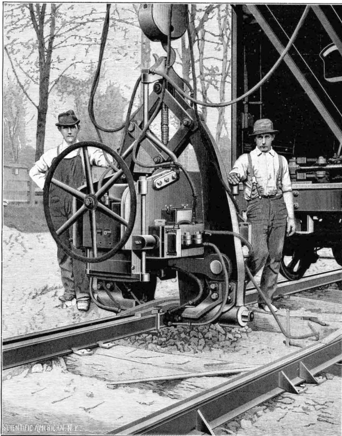
THE ELECTRIC WELDING OF RAIL JOINTS.
