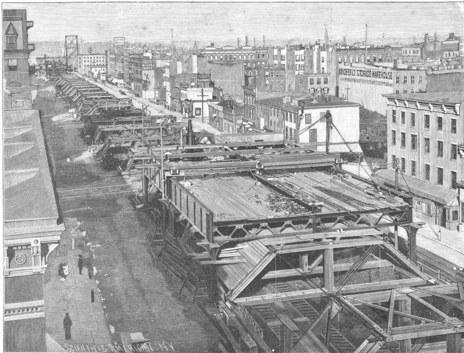
THE PARK AVENUE IMPROVEMENT IN NEW YORK.
