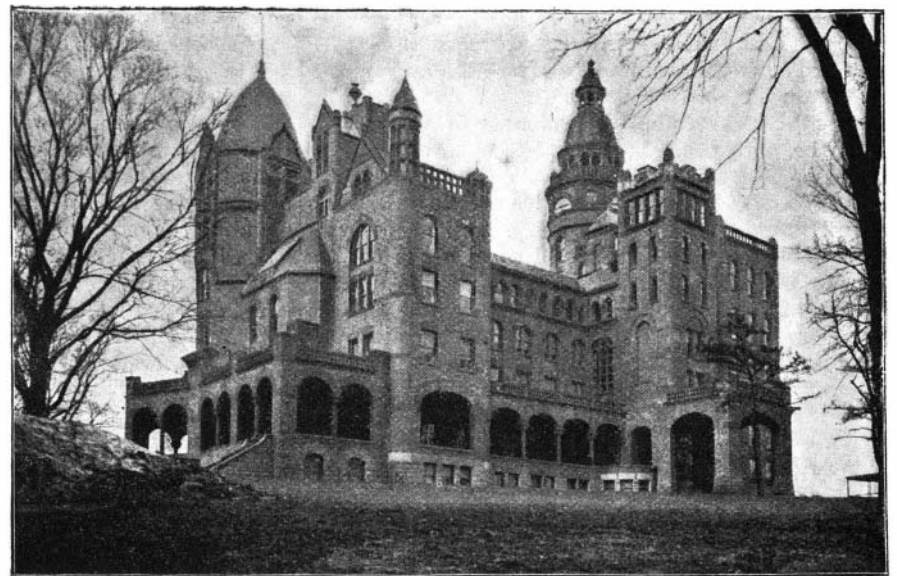
SOUTHEAST ASPECT WITH CORRIDOR.
