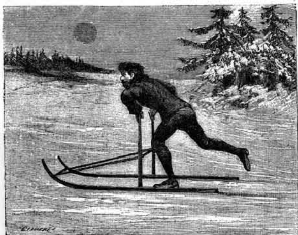
Fig. 2.—METHOD OF USING THE SPARKSTOTTING.
