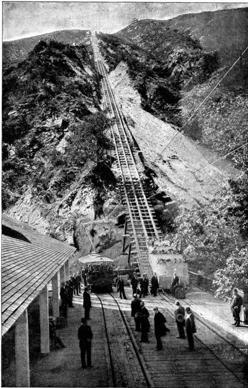
THE GREAT CABLE INCLINE, MT. LOWE RAILWAY, CALIFORNIA.
