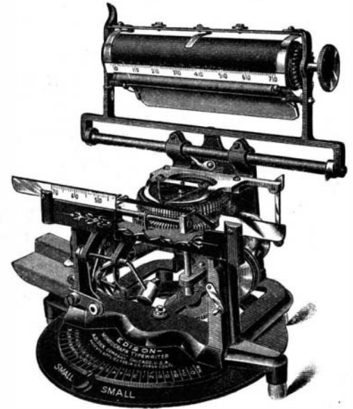
With carriage raised and scale cut away, showing ribbon movement.
