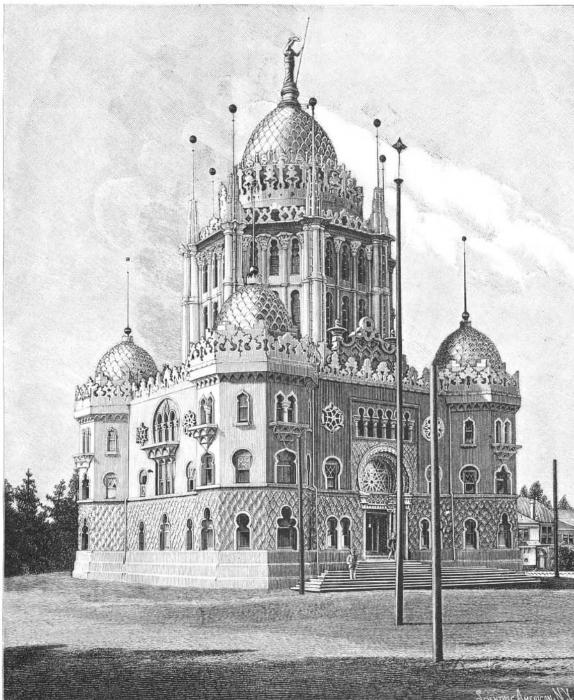
THE CALIFORNIA MIDWINTER FAIR—THE ADMINISTRATION BUILDING.
