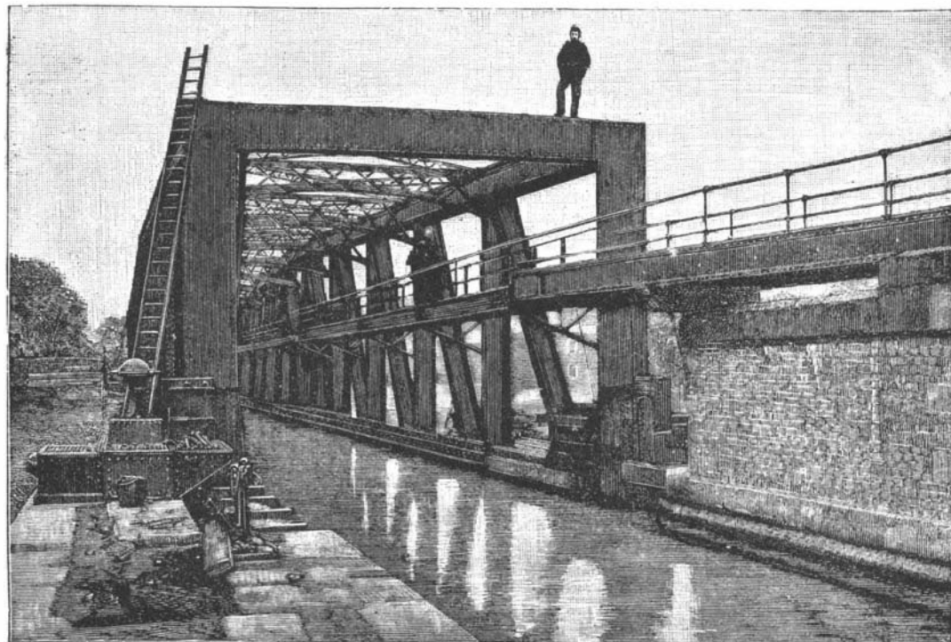
THE MANCHESTER SHIP CANAL—BARTON SWING AQUEDUCT, CARRYING THE OLD BRIDGEWATER CANAL ACROSS THE SHIP CANAL.
