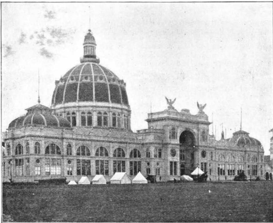
THE GOVERNMENT BUILDING.
