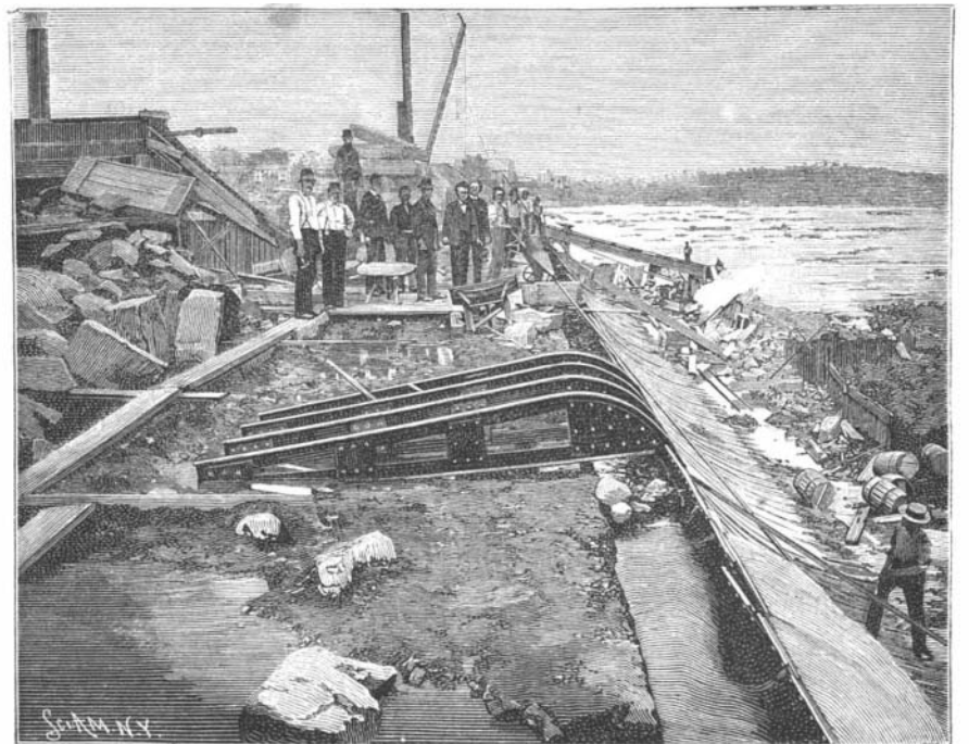
Fig. 2.—THE NEW STATE DAM, COHOES, N. Y.—SHOWING THE TOP FRAME.
