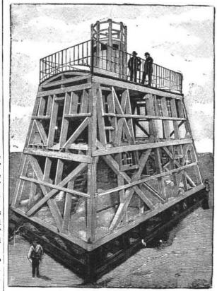
Fig. 1.-FRAMEWORK OF THE JANSSEN OBSERVATORY MOUNTED UPON THE SNOW AT THE SUMMIT OF MONT BLANC.
