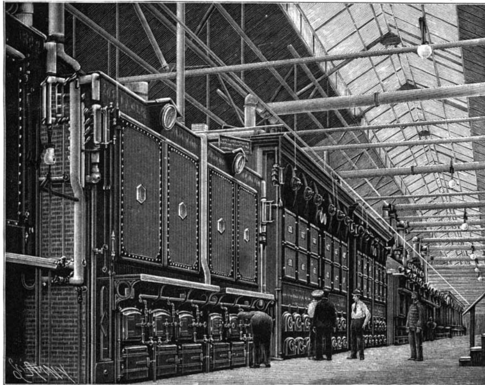
OIL-FIRED BOILERS AT THE GREAT EXPOSITION.
