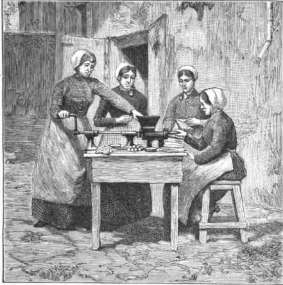
Fig. 7.—FILLING CARTRIDGES WITH EXPLOSIVE GUM.
