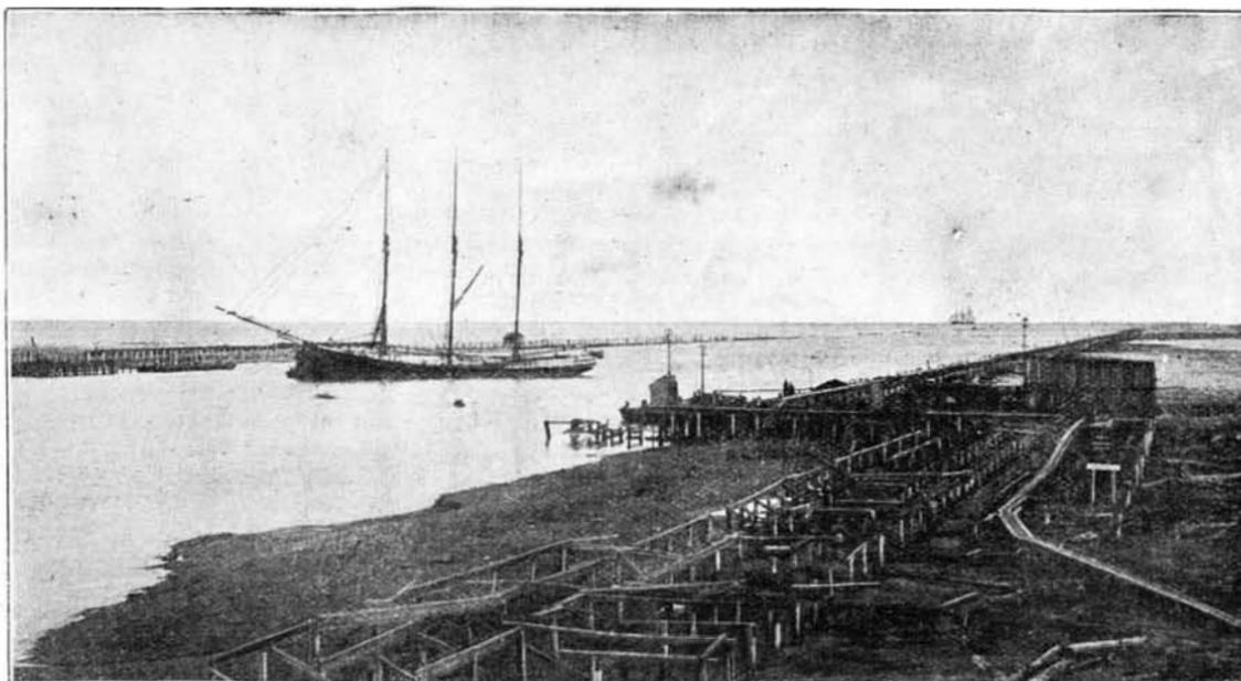
bouches boldly into the Gulf of Mexico in one solid stream, there being no delta formation at its mouth. The current of this great river will rush through the channel made by the jetties, scour away the sand and mud, and thus carry out the design of the engineer by acquiring and maintaining a depth of 20 feet of water over the bar.
