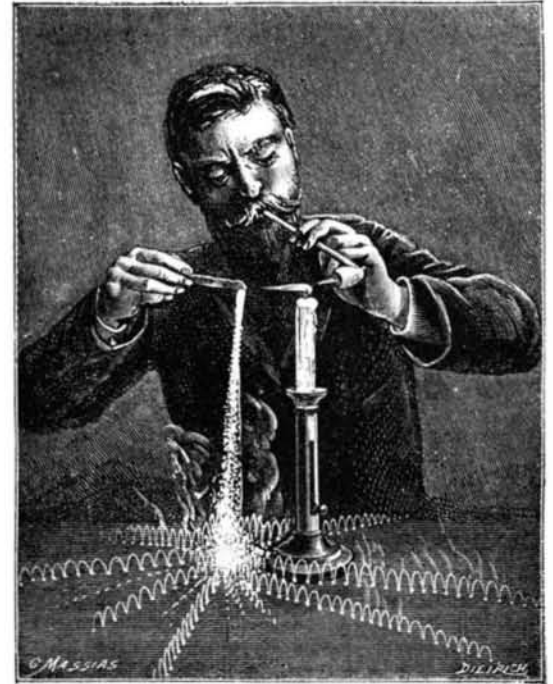
COMBUSTION OF TINFOIL IN THE FLAME OF A BLOWPIPE.
