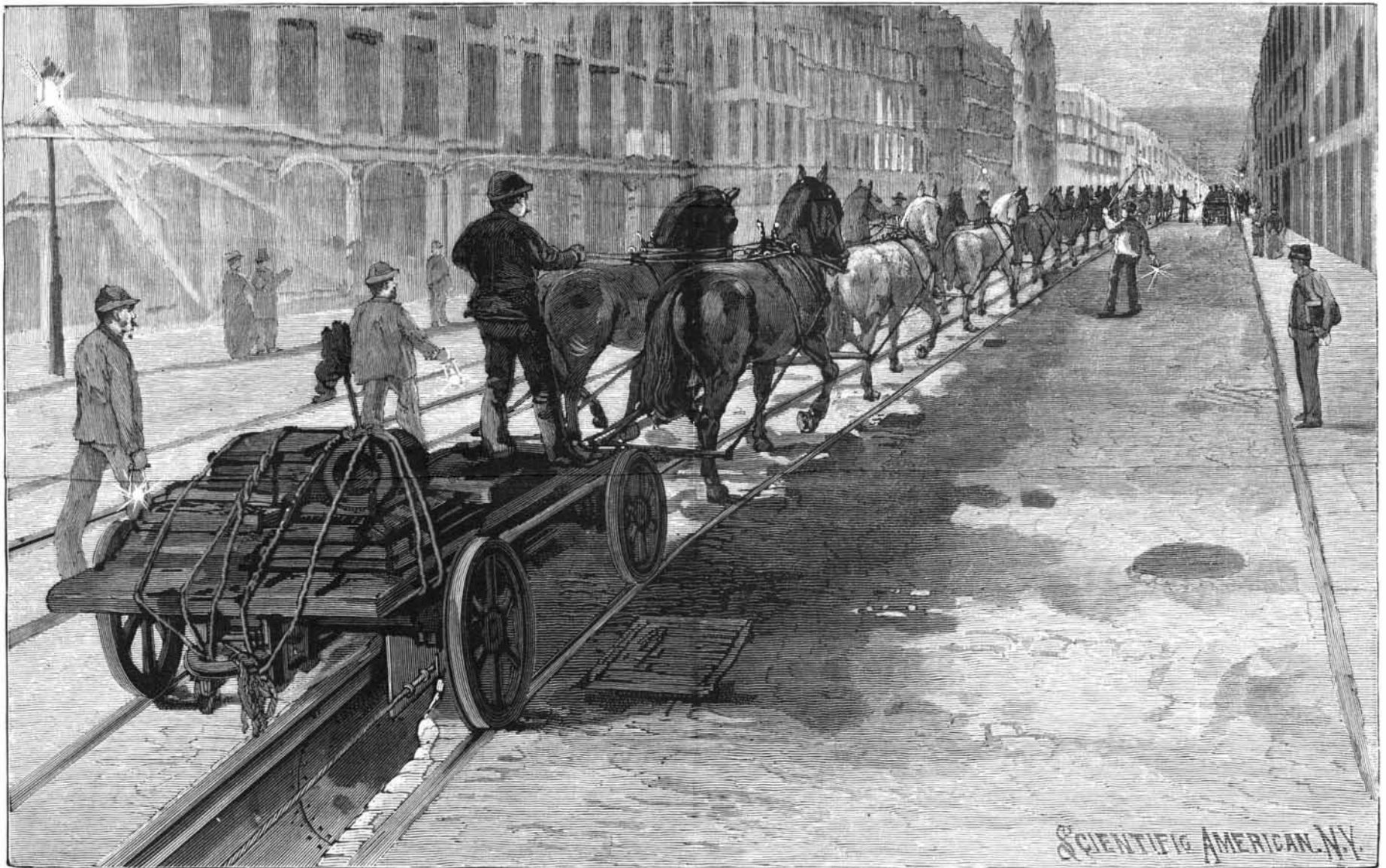
THE BROADWAY CABLE RAILWAY NEW YORK—RUNNING IN THE CABLE.
