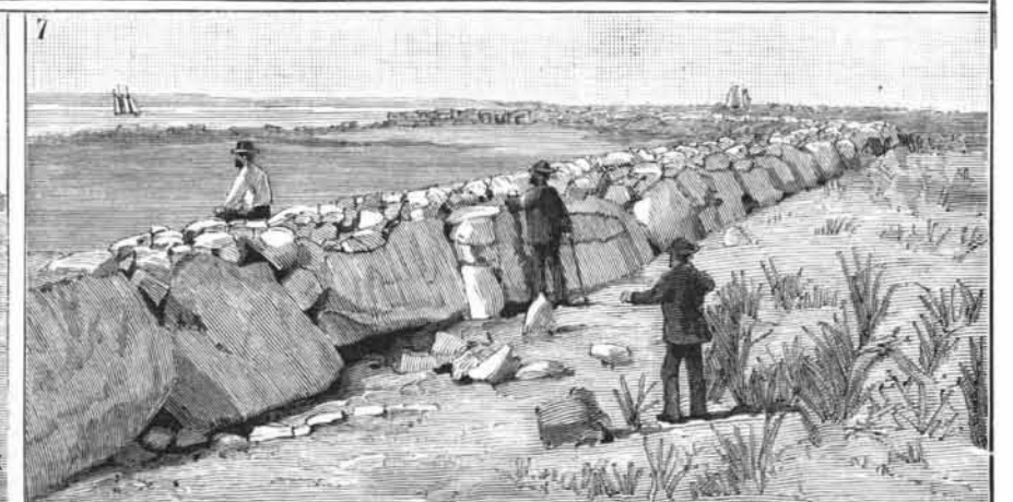
1. Bird's eye view of Boston harbor. 2. Cross section showing retaining wall. 3. Point Allerton. 4. Gallup's Island. 5. Long Island. 6. Sea wall, Lovell's Island. 7. Rubble stone apron, Lovell's Island.
