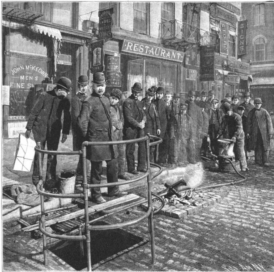
FORCING HOT AIR INTO THE SUBWAYS, NEW YORK.
