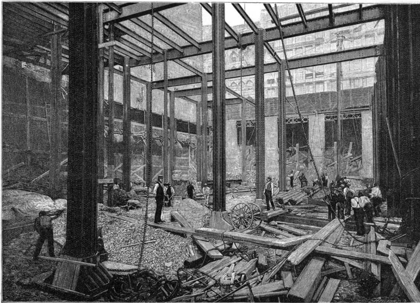
DEEP BASEMENT OF THE BROADWAY R.R. POWER HOUSE, CORNER OF HOUSTON STREET.
