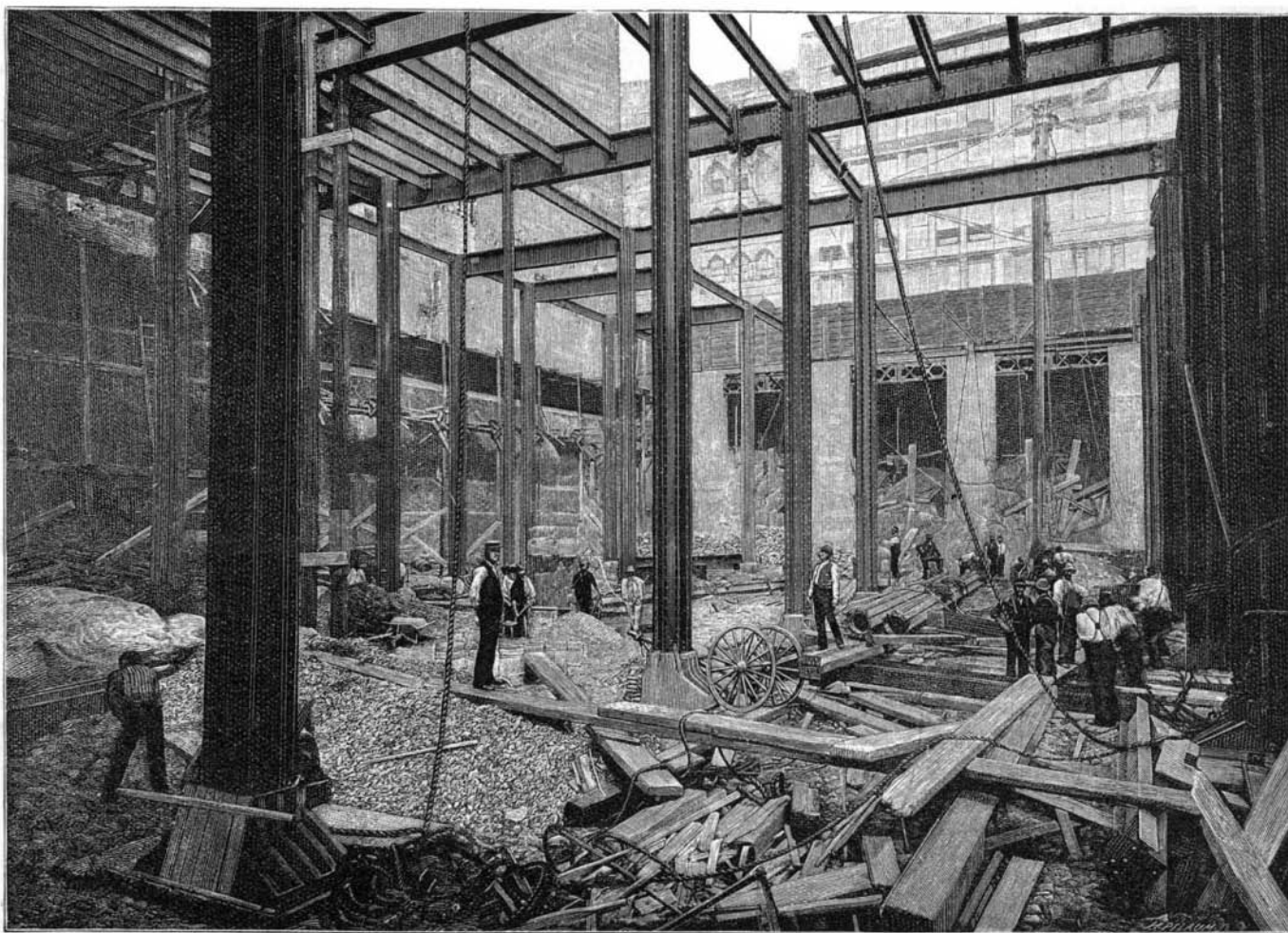
DEEP BASEMENT OF THE BROADWAY R.R. POWER HOUSE, CORNER OF HOUSTON STREET.
