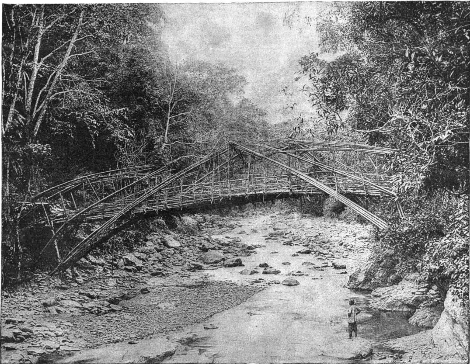
A BAMBOO BRIDGE IN SIKKIM, INDIA.—PLATE BY THE PAPHYROTINT PROCESS.
