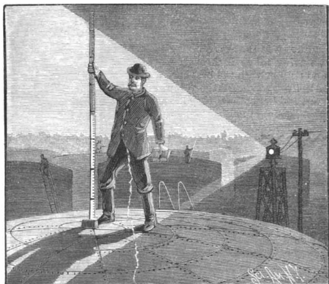
SOUNDING OIL TANKS AT NIGHT.
