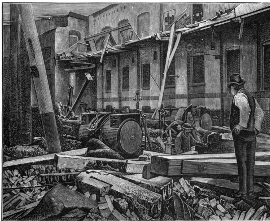
BURSTING OF FLYWHEEL—AMOSKEAG MILLS.
