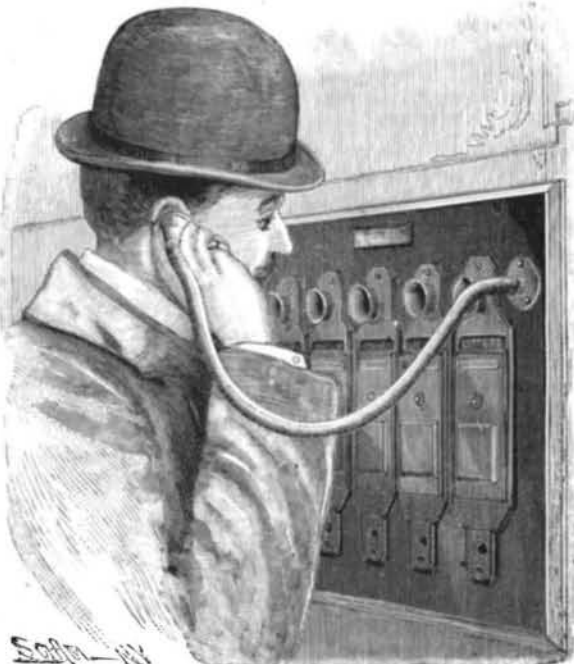
SCHLUCHTNER'S SPEAKING TUBE—USE IN A VESTIBULE.]
