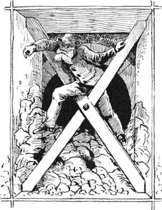
CHIEF ENGINEER HOBSON BREAKING THROUGH FROM CANADA TO THE UNITED STATES UNDER THE ST. CLAIR RIVER.
