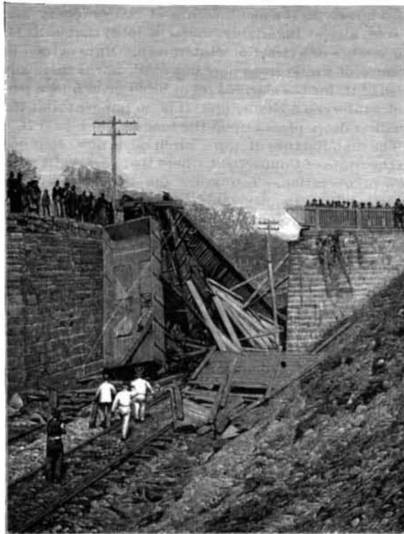
A SINGULAR BRIDGE ACCIDENT.
