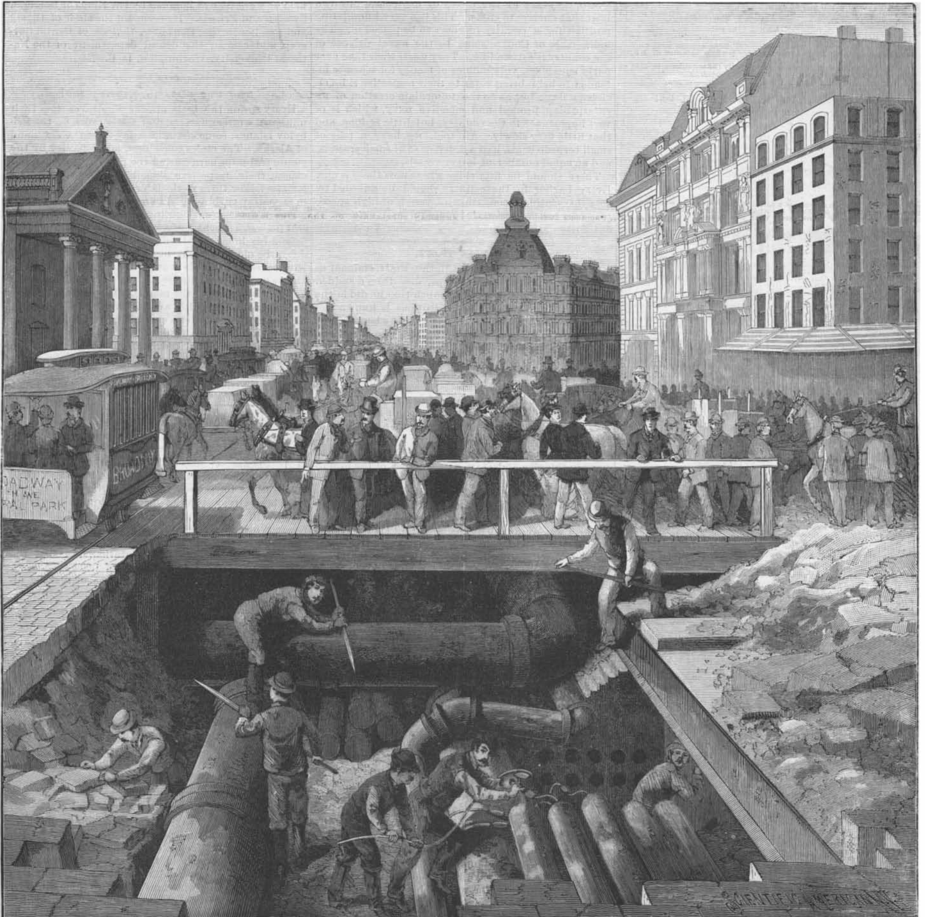
THE BROADWAY AND SEVENTH AVENUE RAILROAD—CLEARING OBSTRUCTIONS FROM THE LINES OF THE CONDUITS.
