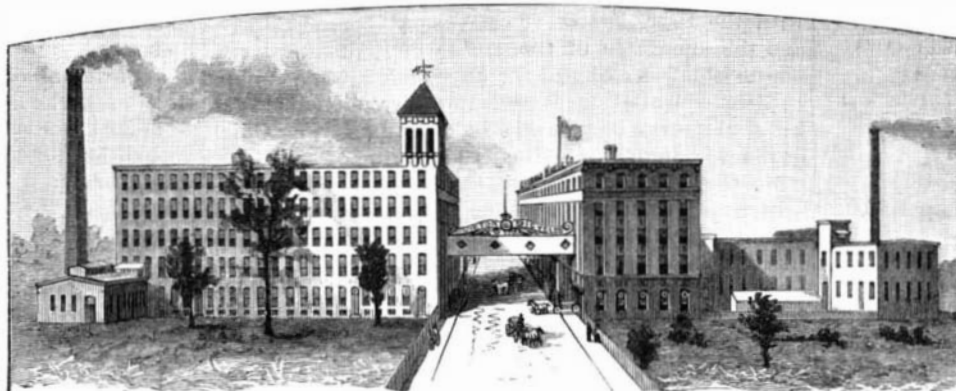
GENERAL VIEW OF THE WORKS AT CHICOPEE FALLS MASS.
